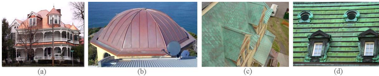
Figure 22: (a) A newly built copper roof on a building. (b) Dark-brown tarnish layer gradually turns into red-brownish color. (c) and (d) Green patina development aging 25 years or more.
