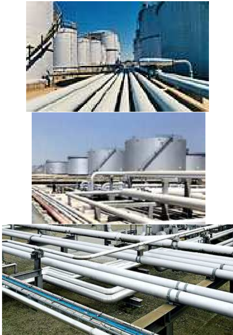
Fig. C.7. Oil and Gas Switches
