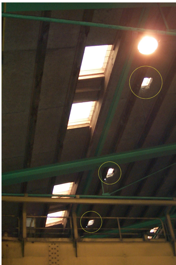
Figure 10.2: Ceiling with three of the four holes for the cameras marked with circles. The fourth hole is covered by the crane.
